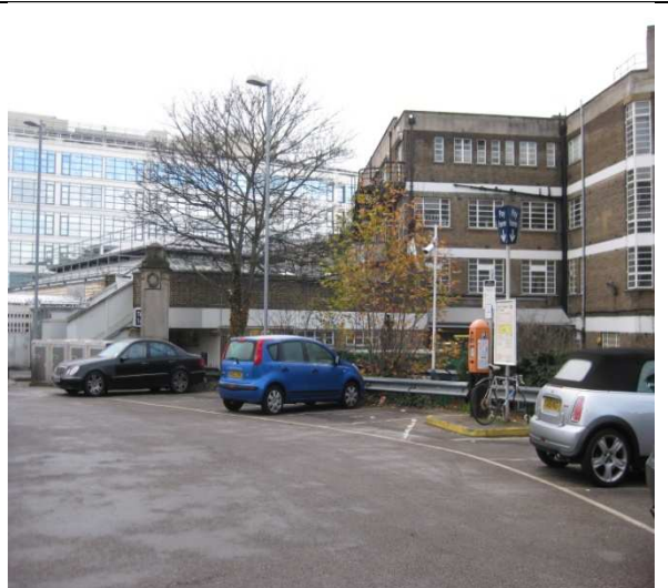
PR11 – Station car park
